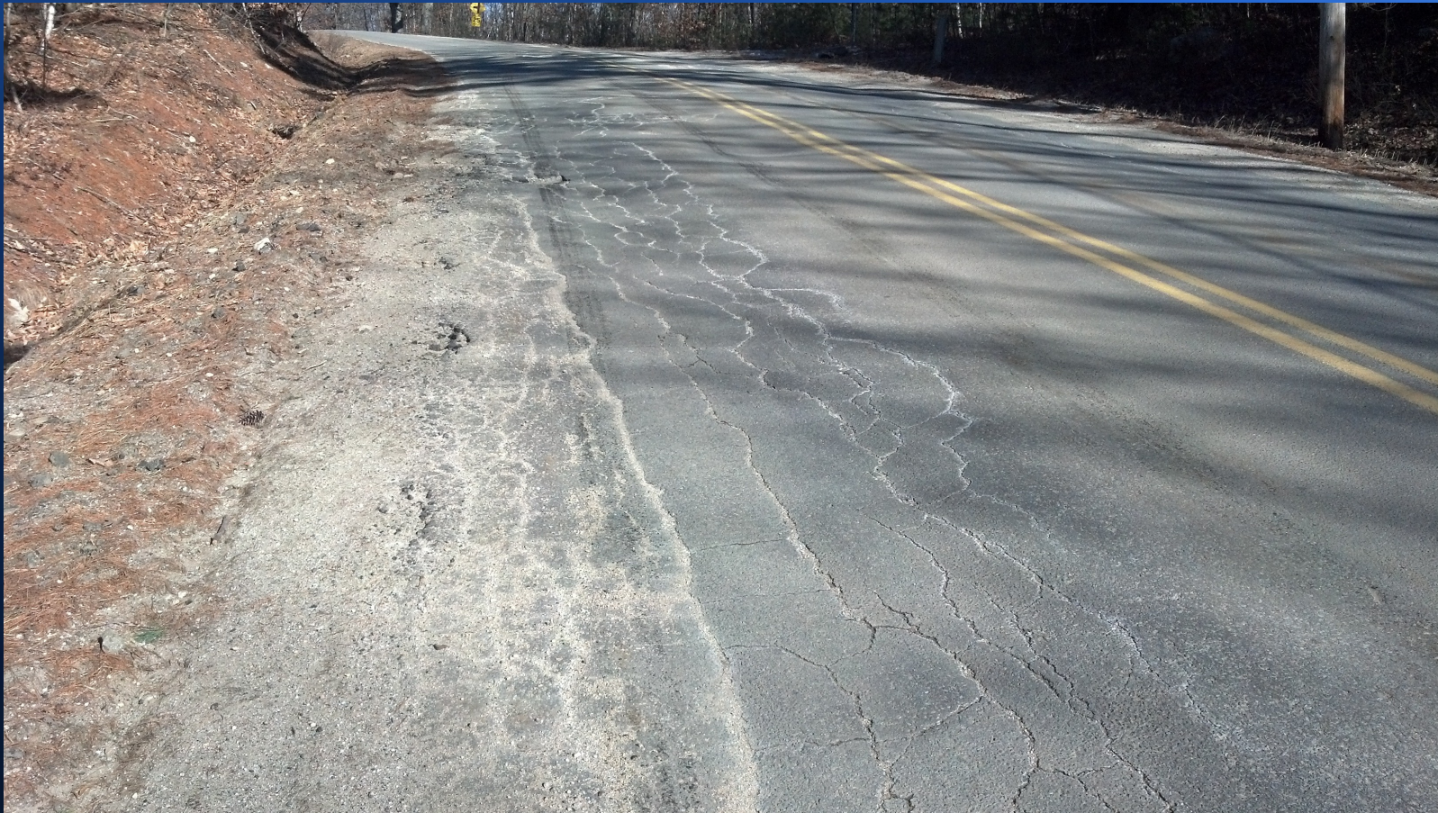
“Alligator” Cracking and Shoulder Deterioration
