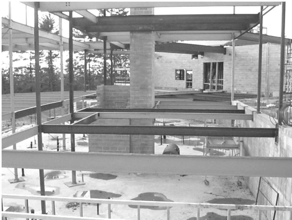
The Raymond Elementary School evolves as structural steel is put in place.
