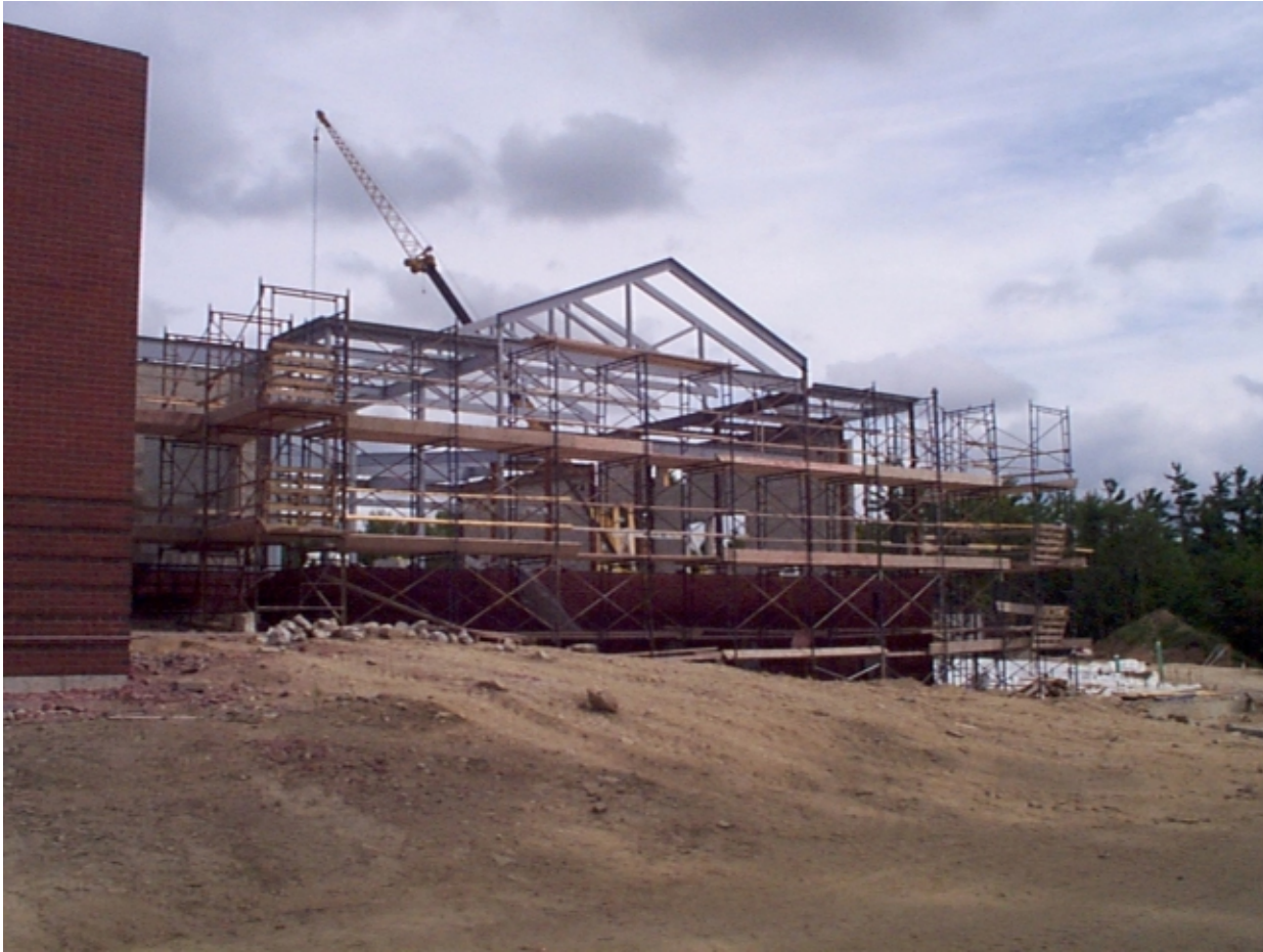
The Media Center at the Raymond Elementary School takes shape.
