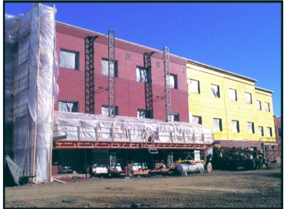
The new Raymond Elementary School gets its brick facing.
