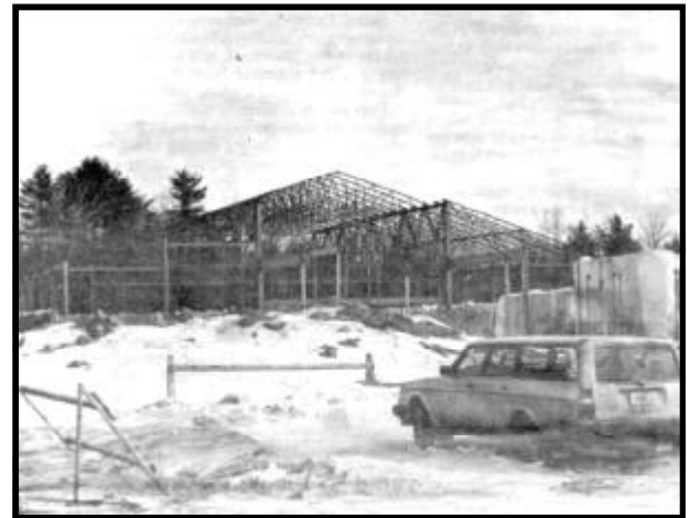
Building the gym in 1988.
