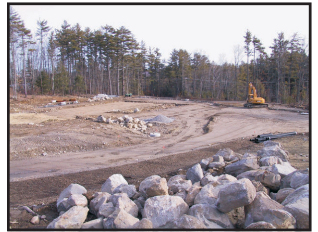
Site of the new firestation where the water line will terminate.
