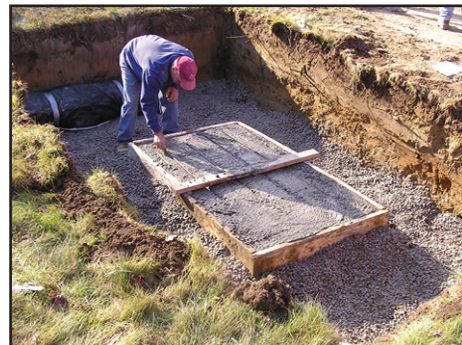
Bob Flynn working the concrete.
