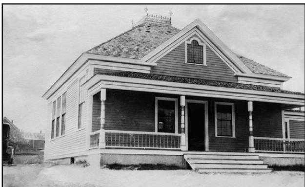
East Raymond School, ca. 1925. Picture provided through the courtesy of the Maine Memory Network of the Maine Historical Society
