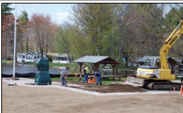
Raymond Public Works spreading loam - photo by David McIntire
