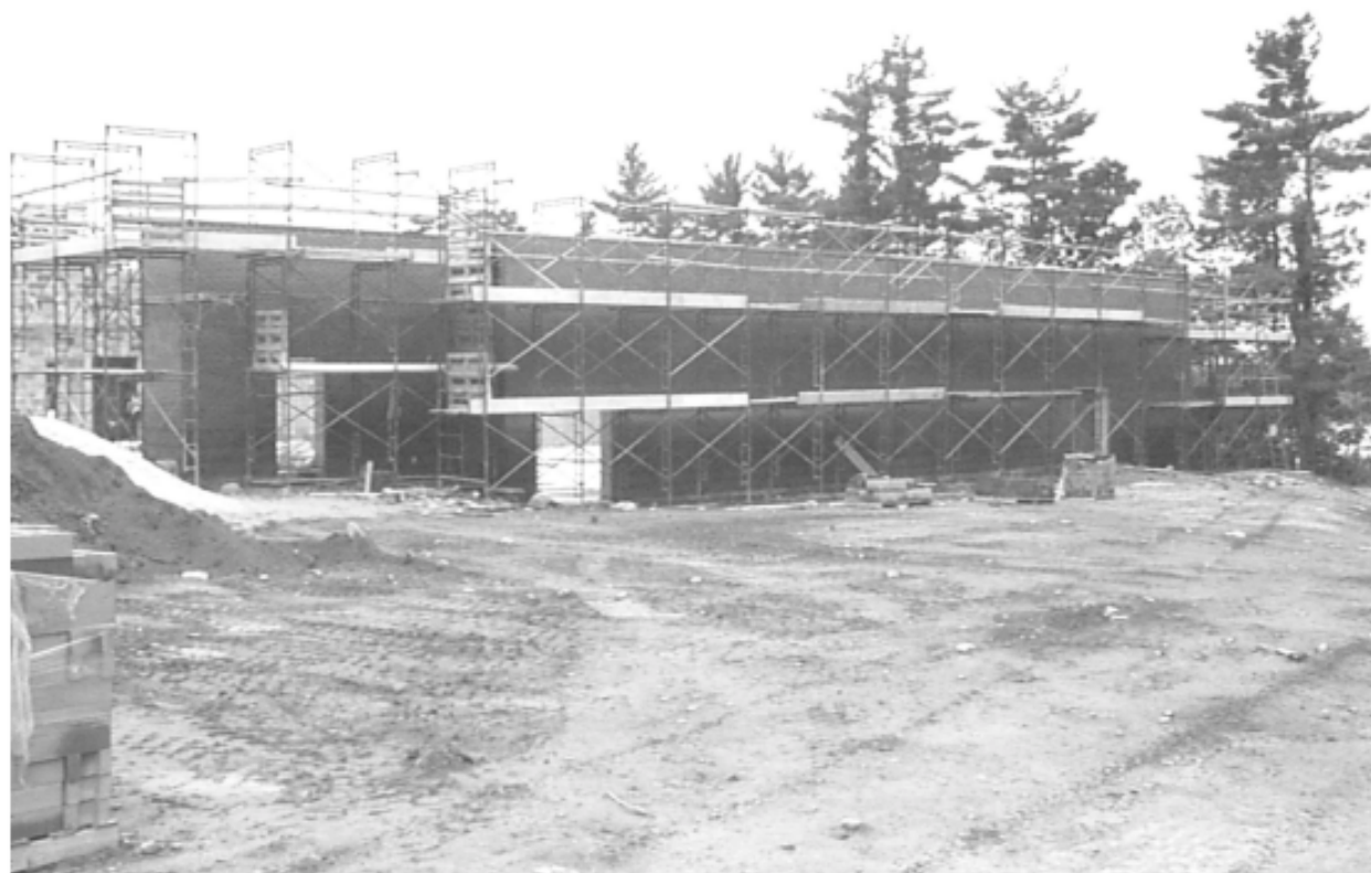
Bricks and Mortar Being Applied to the New Elementary School
