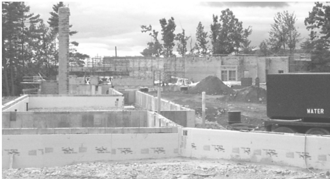
Foundation Work Nears Completion at the New Elementary School on August 22, 1999
